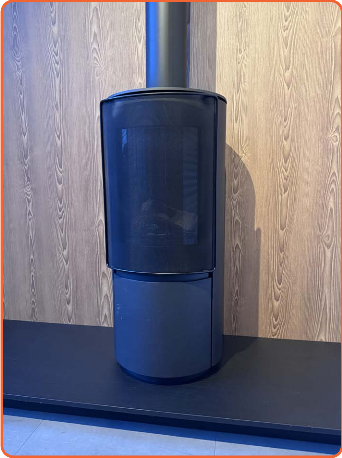
Figure 5.10 | Safety screen installed
